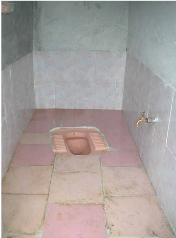
Photo 3 Inside the toilet, use tiles for easy maintenance
