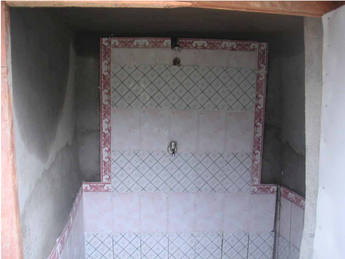
Photo 5 Inside the bathroom
