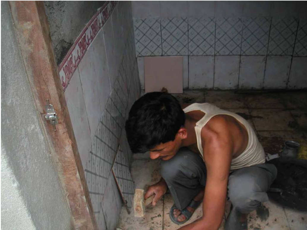
Photo 1: It was really hard to build a toilet and bathroom.
